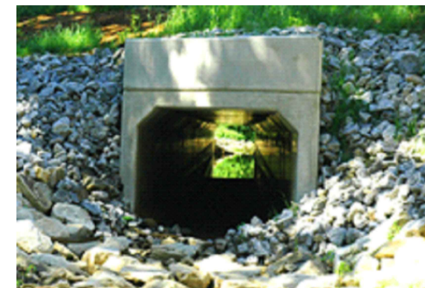
CULVERT OUTLET @ DISCHARGE POINT
